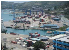
Existing Port of Port Moresby
